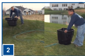
2 Place skimmer and biological filter into position.
