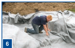
6 Install the liner and underlayment.
