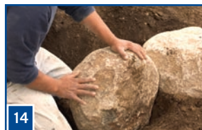
14 Build the retaining wall.
